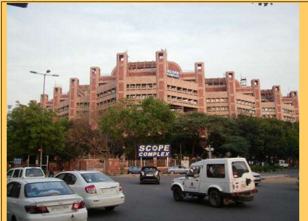
Scope Building di Raji Rewal ( 1989)
