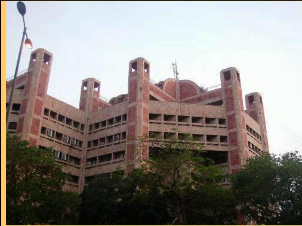
Scope Building di Raji Rewal (1989)
