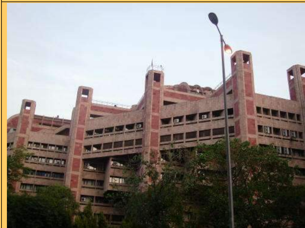
Scope Building di Raji Rewal (1989)
